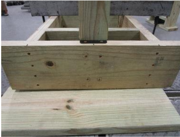
Photo No. 5 Mock Deck Fabrication
