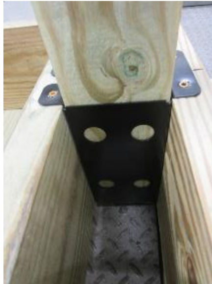
Photo No. 1 Installed Post Mount Bracket
